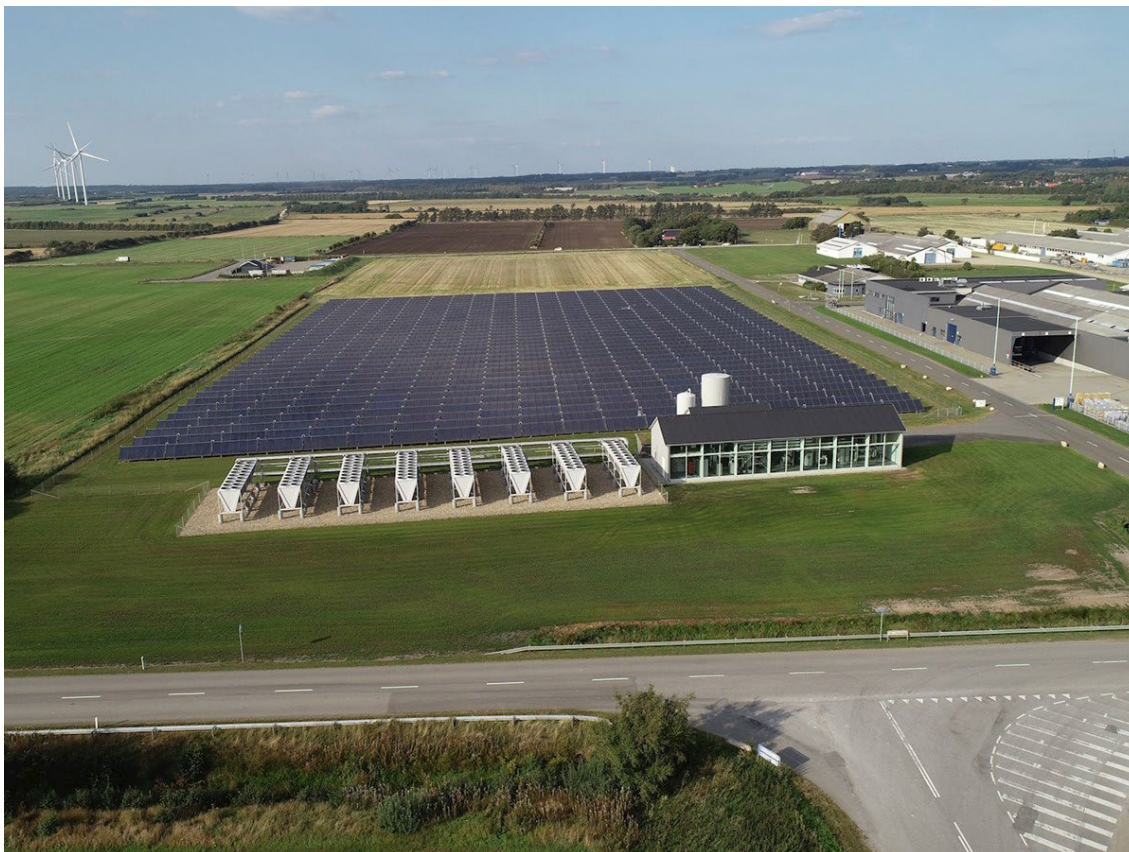
Slika 14: Lem district heating plant
